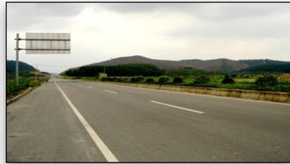
Paved highway near Fuwan
